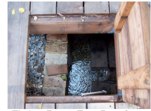
Timber Frame Trap Door for Spring Head
